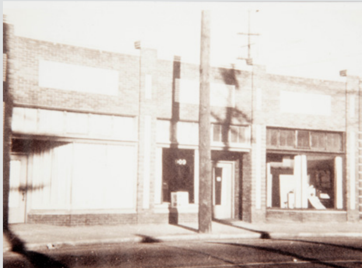
The building at 909 West Jefferson Blvd. (Home of the Los Angeles School of Optometry from 1936 to 1948).
