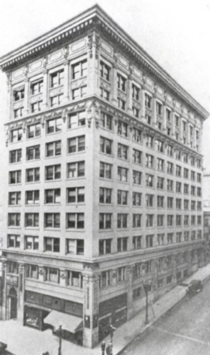
The Wright & Callender building in Los Angeles (Home of the Los Angeles School of Optometry from 1922 to 1928).
